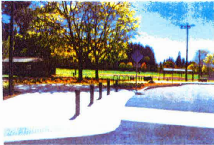
The combination of sloped corner curbs and bollards may be incorporated with crosswalks within the commercial areas.
