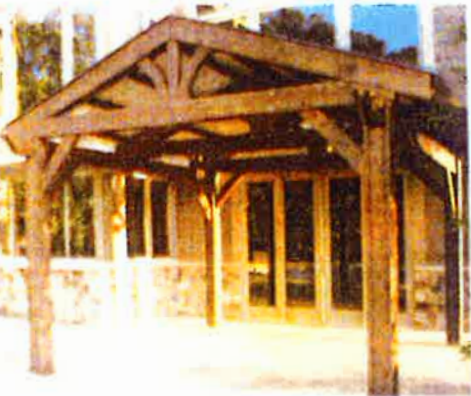
The wooden beams of the above arbor imitate the half timbering, used throughout England. This method of support shall be applied to all applicable shade structures.
