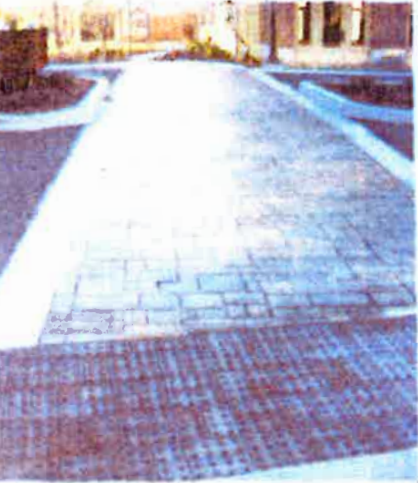
This is a great example of an approved ADA crosswalk using stamped and stained concrete.
