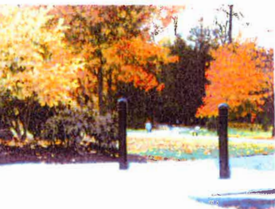
Bollards at trail intersections not only discourage cars from utilizing trails, but also provide pedestrian safety in the event an accident occurs at this location.
