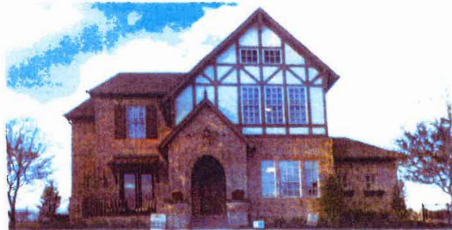
In this image the half timbering and multi-paned windows are the highlighted Texas Tudor elements to replicate.
